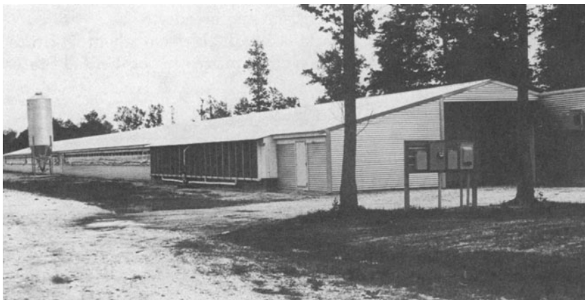
FIG. 11.2. A broiler breeder house. Courtesy of Perdue, Inc.
