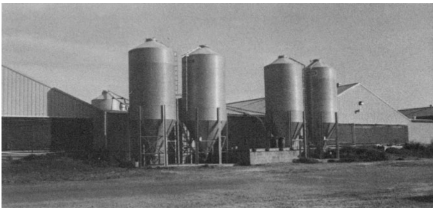
FIG. 8.1. Feed storage bins in a modern poultry operation. Feed is conveyed directly from the trucks to the bins and then by automatic feeders to the chickens.
