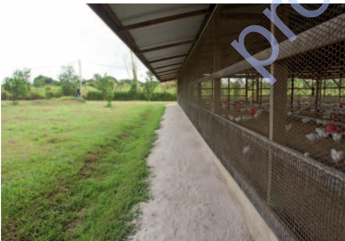
You can restrict the influx of direct sunlight with a roof that extends well beyond the edge of the building. When building a new poultry house, make sure the length of the house runs east-west. This is another way to restrict light influx at noon.
