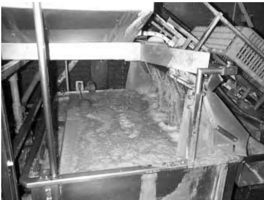
Fig. 6.6 Drawers leaving the soak tank to enter the main wash module (bottom corner only visible in top left of photograph). Water carried over by the drawers and the drainage water from the wash booth fall back into the main water tank via a run-down screen. The ballcock controlling the make-up water is visible near the centre of the photograph.
