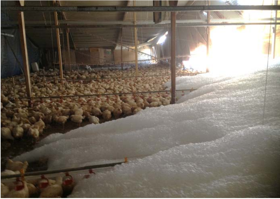
Figure 17.1 Photograph showing the delivery of nitrogen-filled high expansion foam to cull broiler chickens in the United Kingdom. The cull was required due to the rearing building becoming structurally unsafe following a roof collapse.
