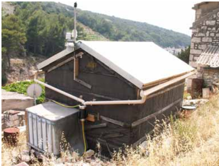
Figure 3. The house in Salbunara bay, NW of Biševo Island. The 15.1 m 2 roof has its symmetry axis oriented east (left)-west (right). Sea is on the west side. (Photo D. Beysens).
